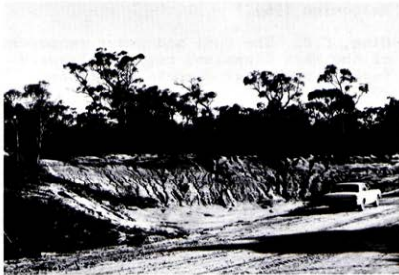
Erosion on the sides of a gravel pit in the Holey Plains Block
