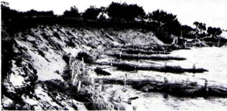
Control of wave erosion following destruction of shoreline vegetation by saline water
