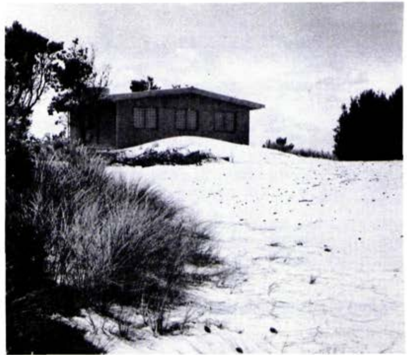
Wind erosion around a house built on the crest of a foredune
