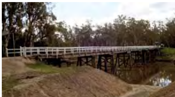
Figure 7.4 Stewarts Bridge was constructed across the Goulburn River at Kanyapella in 1879.
