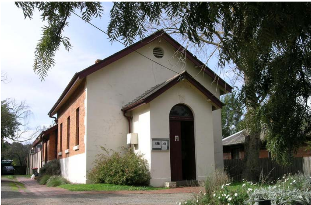
Figure 6. Eltham Court House, designed by the Public Works Department architect Alfred T. Snow, and constructed in 1860. The court house retains many intact early features including the use of handmade bricks, simple decoration, roof trusses, timber ceiling boards, original windows, doors and associated hardware and a collection of court furniture. The court house forms part of an important early justice precinct, with the 1860s police station and stables located next door. (DSE image)
