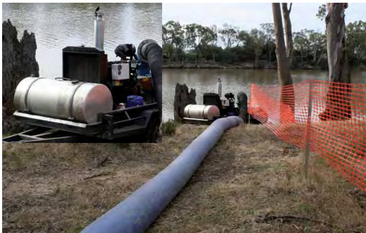
Figure 15.15 Pumping structures for environmental flows directly from river.
