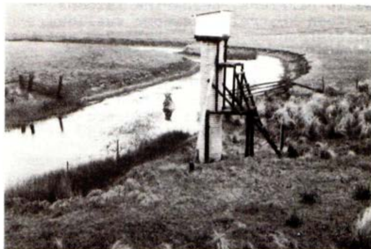
Stream-gauging station on Muston Creek.
