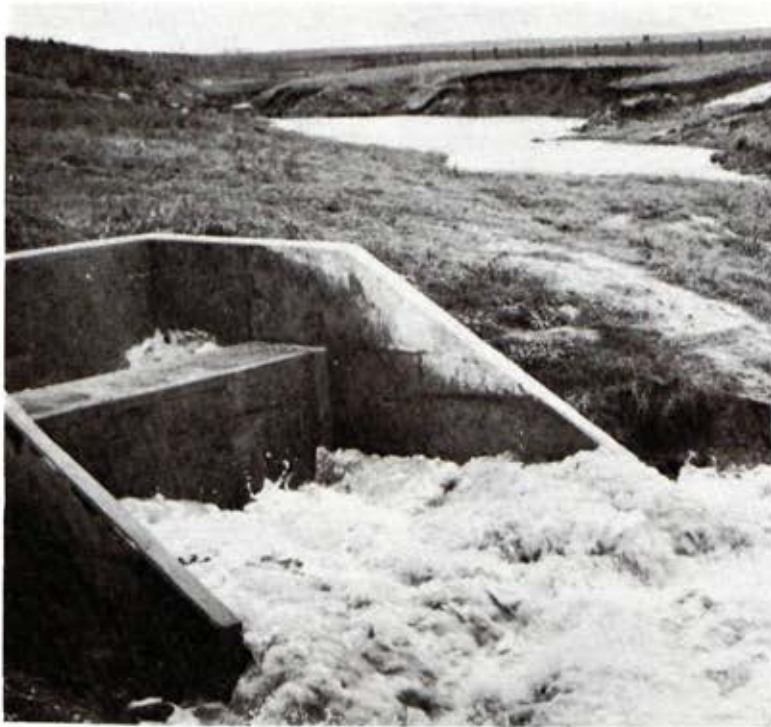
Prevention of flooding: The Woady Yaloak diversion channel outfall.
