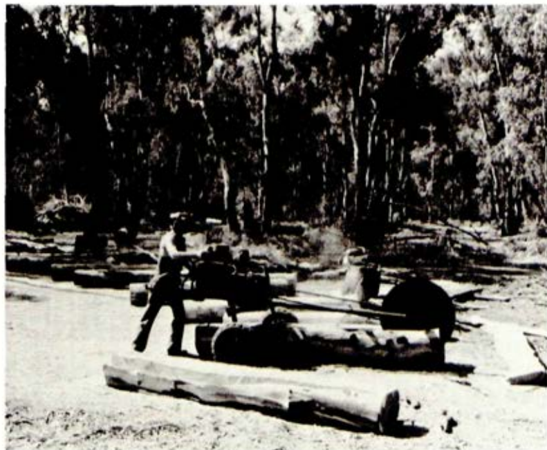
Sleepers being cut using a barrow saw
