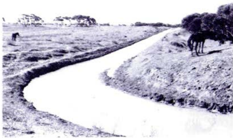
A typical stock and domestic water supply channel
